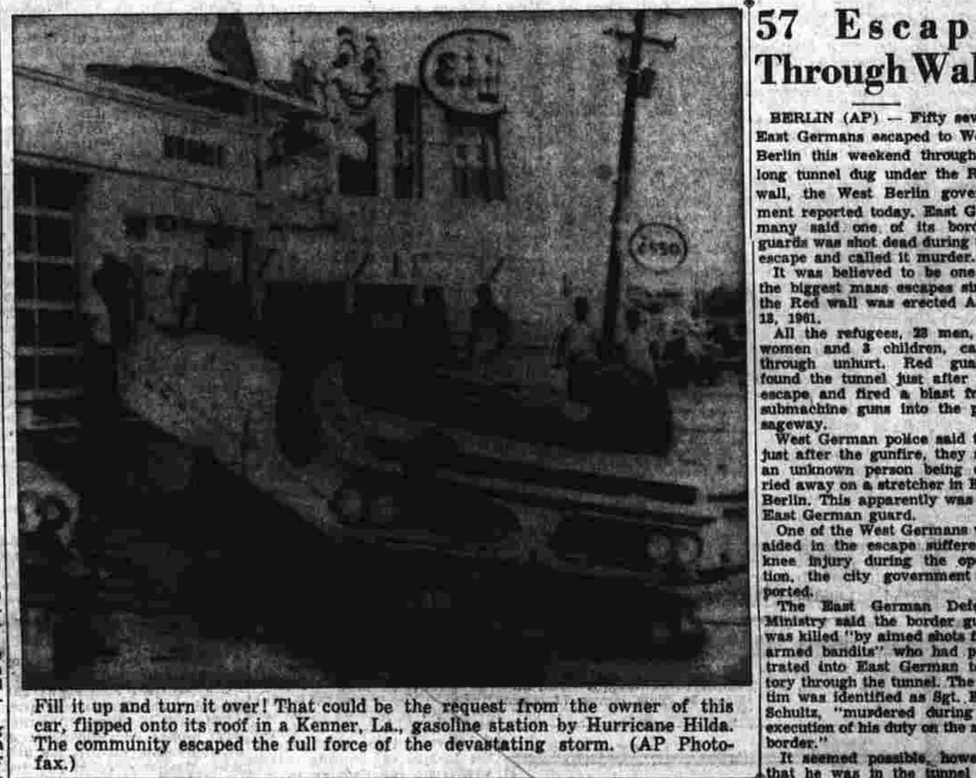
Fill it up and turn it over! That could be the request from the owner of this car, flipped onto its roof in a Kenner, La., gasoline station by Hurricane Hilda. The community escaped the full force of the devastating storm. (AP Photo-fax.)
